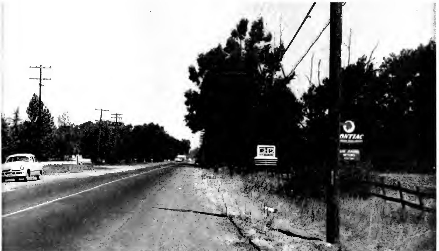
Pacific Avenue in 1950, prior to reconstruction under the Federal Aid Secondary Highway Program
